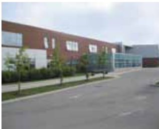
At the École Secondaire Jeunes Sans Frontières in Mississauga, Ontario, 104,700 ft 2 (31,900 m 2 ) of 5/8 in. RAUPEX O 2 Barrier pipe were installed in a concrete-embedded, slab-on-grade design, using a counterflow spiral pattern to promote even surface temperatures.
