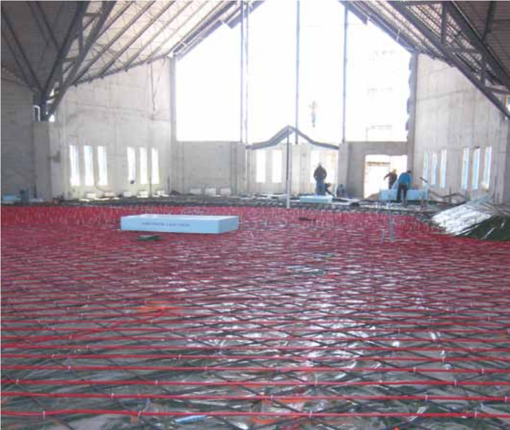
9,000 ft (2,740 m) of RAUPEX O 2 Barrier pipe installed.
