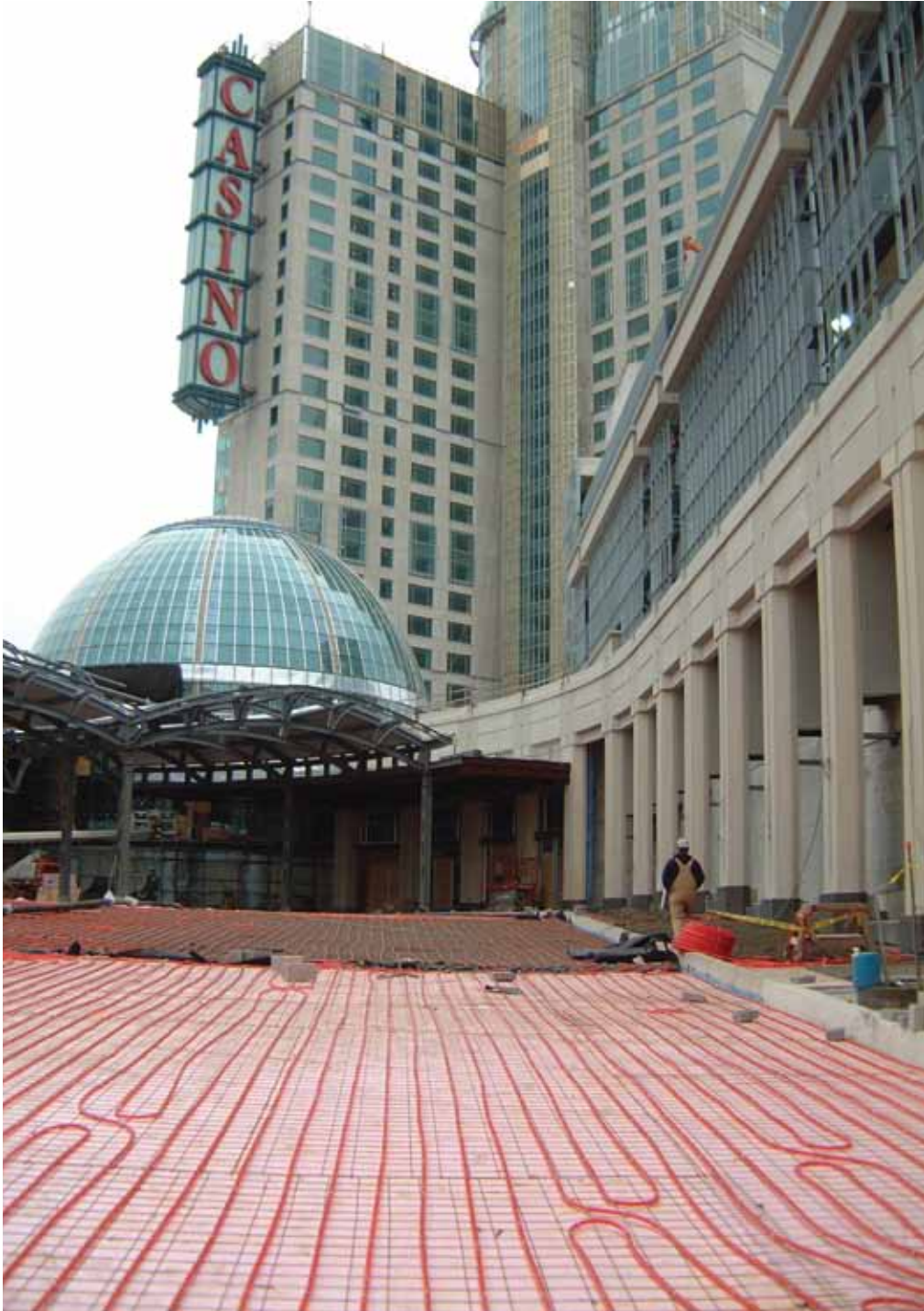
125,000 ft 2 (11,600 m 2 ) of snow and ice melting system in parking lots and walkways at Fallsview ® Casino Resort, Ontario, ensures year-round pedestrian safety and vehicle access.
