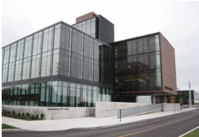
REHAU SIM system will clear pedestrian pathways around the Vaughan City Hall in Ontario.
